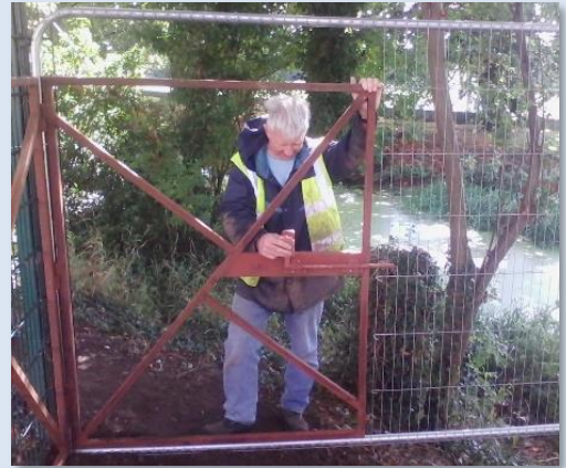
Gate frame being fitted
