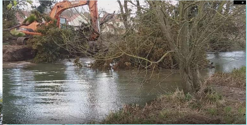
Digger of destruction!
