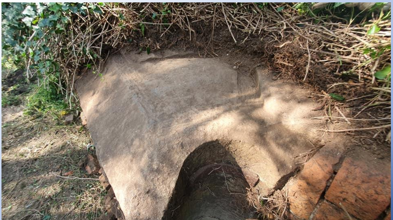
Similar recess on opposite existing wall
