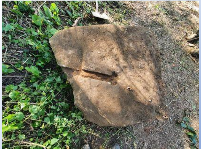
Collar-retaining recess cut into towpath side
