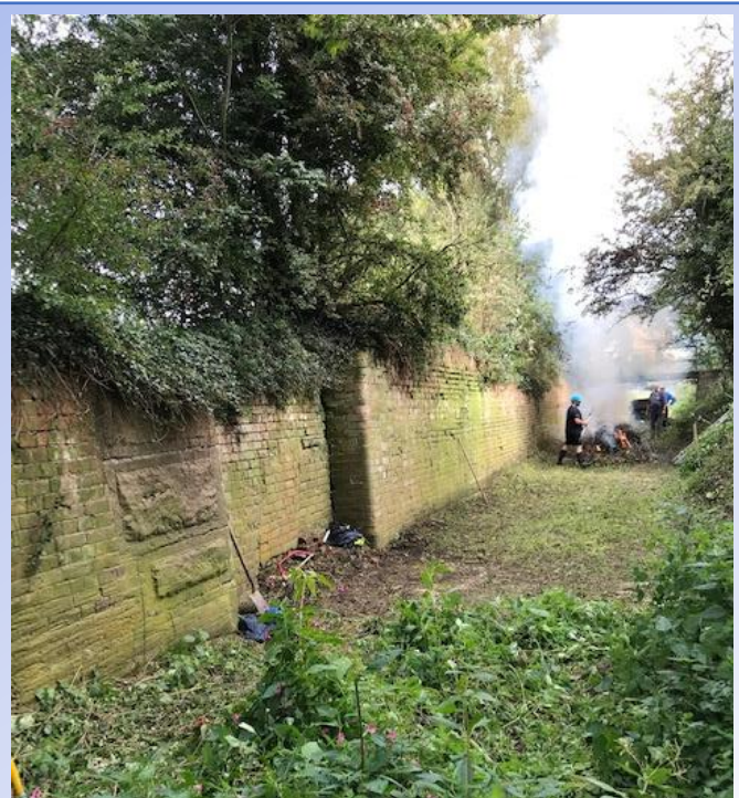
Gate recess showing beautifully dressed stone blocks forming the quoin
